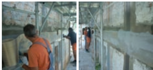
Figure 20. Strengthening of the ring curb beams using steel fiber sheets.
