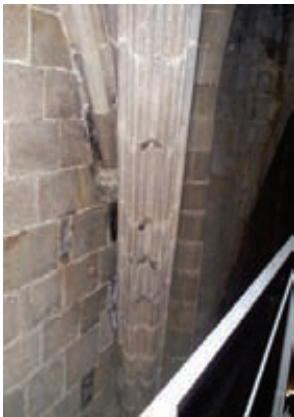
Fig. 6. Arch with mortar expelled in Santa Maria del Mar (left) and microscope picture of mortar showing soot contamination (right)
