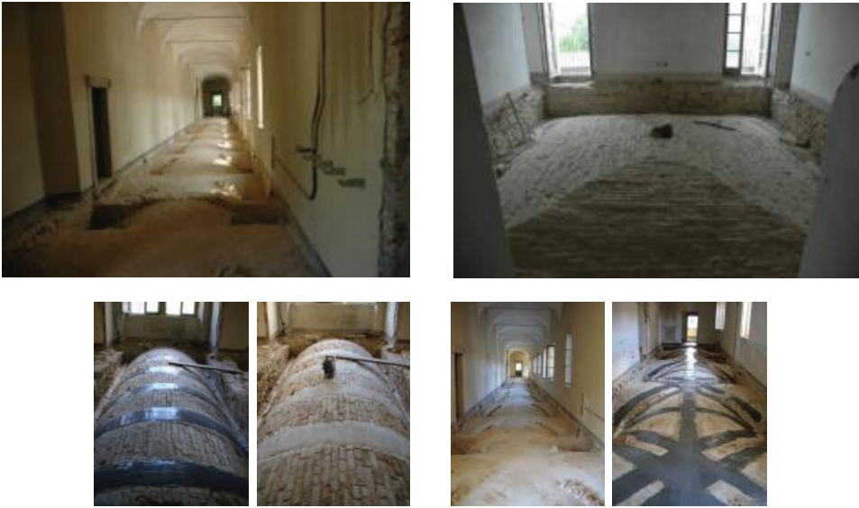
Figure 7. Strengthening of the different types of vaults.
