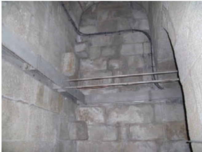
Fig. 3 General sight of the reinforcement system
