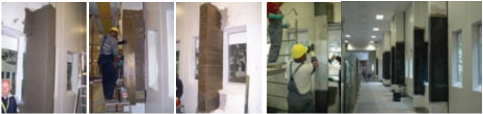
Figure 13. Overview of columns strengthening phases.
