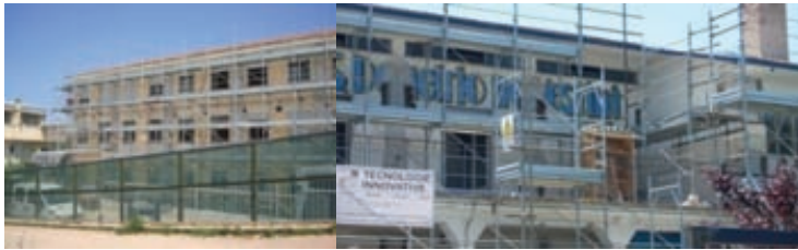
Figure 17. Overview of the damaged San Demetrio Primary School.
