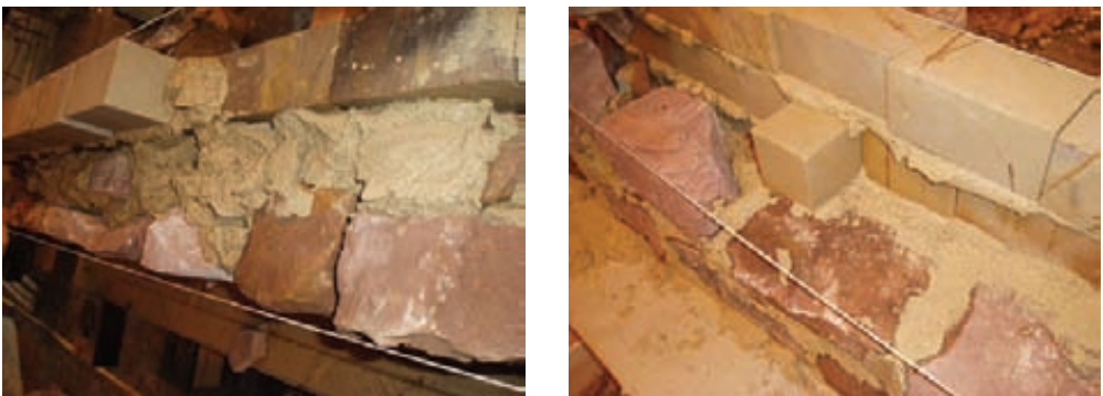
Fig. 5. Detail of the leaves during construction.
