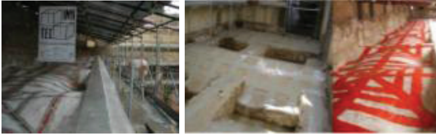
Figure 3. Retrofit of the masonry barrel and vaults with unidirectional GFRP sheets.
