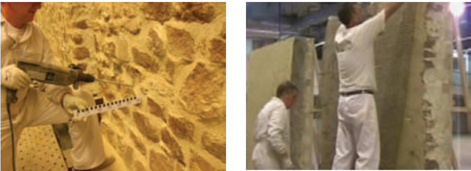
Fig. 6. TRM reinforcement process: Drilling holes (left), placement of basalt textile (right).
