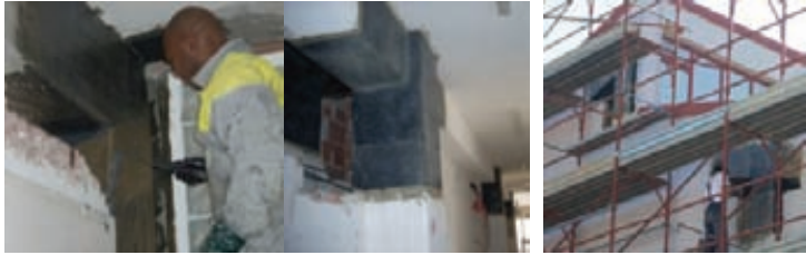
Figure 16. Retrofit phases for the beam-column joint repair
