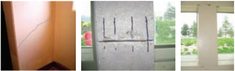
Figure 11. Damaged columns.
